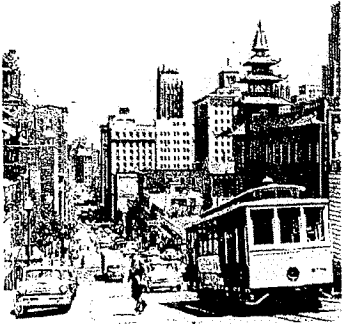
Cable Car on California Street
